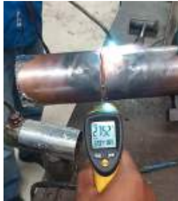
Gambar 3. 4 Proses Preheat
