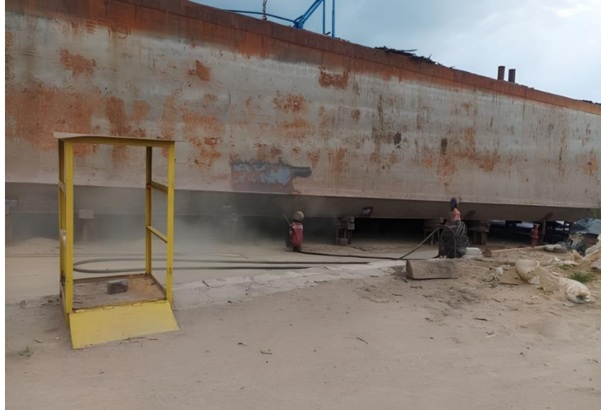
Gambar 2. 2 Proses Sandblasting (Yamin & Yasim, 2023)
