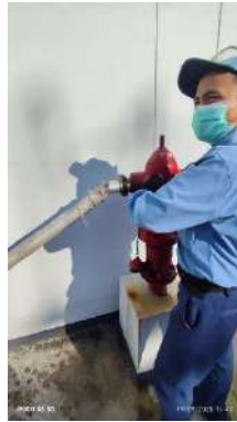
Gambar 2. 2 Pillar Hydrant
