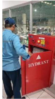
Gambar 2. 4 Inspeksi Hydrant
