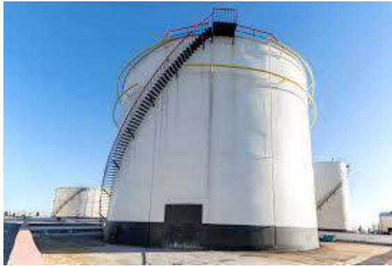
Gambar 2.3 Aboveground Tank Sumber: Admin, 2019
