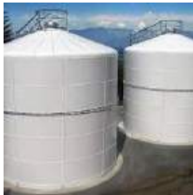
Gambar 2.5 Self Supported Cone Roof Tank Sumber: Jarić et al., 2025
