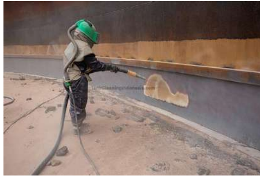
Gambar 1. 1 Ilustrasi sandblasting di Galangan Sumber : https://www.google.com/sandblasting
