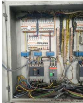
Gambar 2.2 Sub Distribution Panel (Dokumentasi Pribadi)
