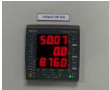
Frequency Sumber ke 1 = 50,7 Hz
