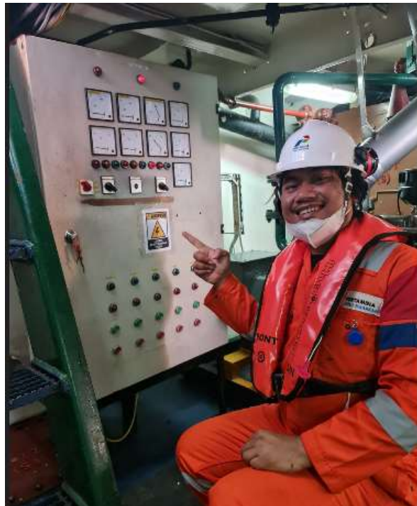
Gambar 3. 2 Panel listrik shore connection di kapal MRP 19
