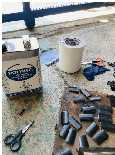
Gambar 4.14 Proses Wrapping
