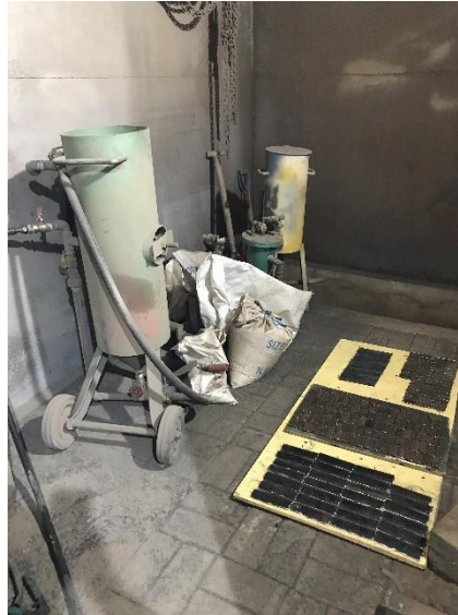
Gambar 4.4 Proses Persiapan Sandblasting
